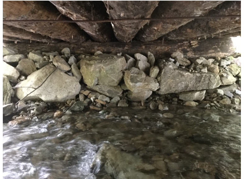
Right Bank Abutment when facing downstream
