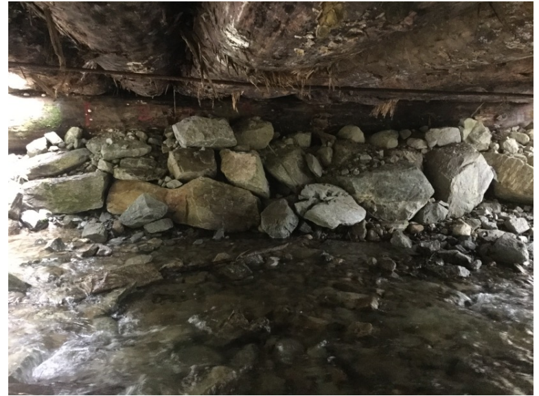
Left Bank Abutment when facing downstream
